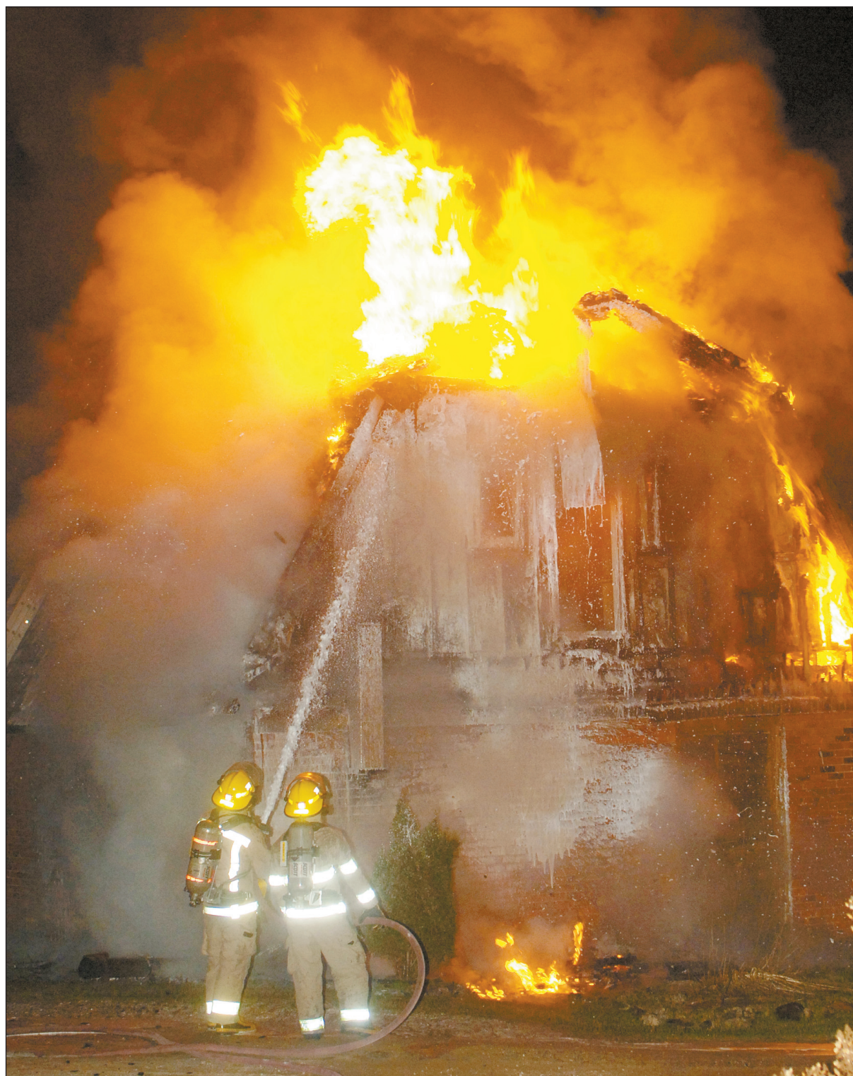
Approximately 30 Halton Hills firefighters worked throughout the evening and into the early morning Wednesday to extinguish this house fire on Sixth Line. Damage is estimated at $150,000 and the suspected cause of the blaze is a design deficiency in a wood-burning stove or how it was installed.
