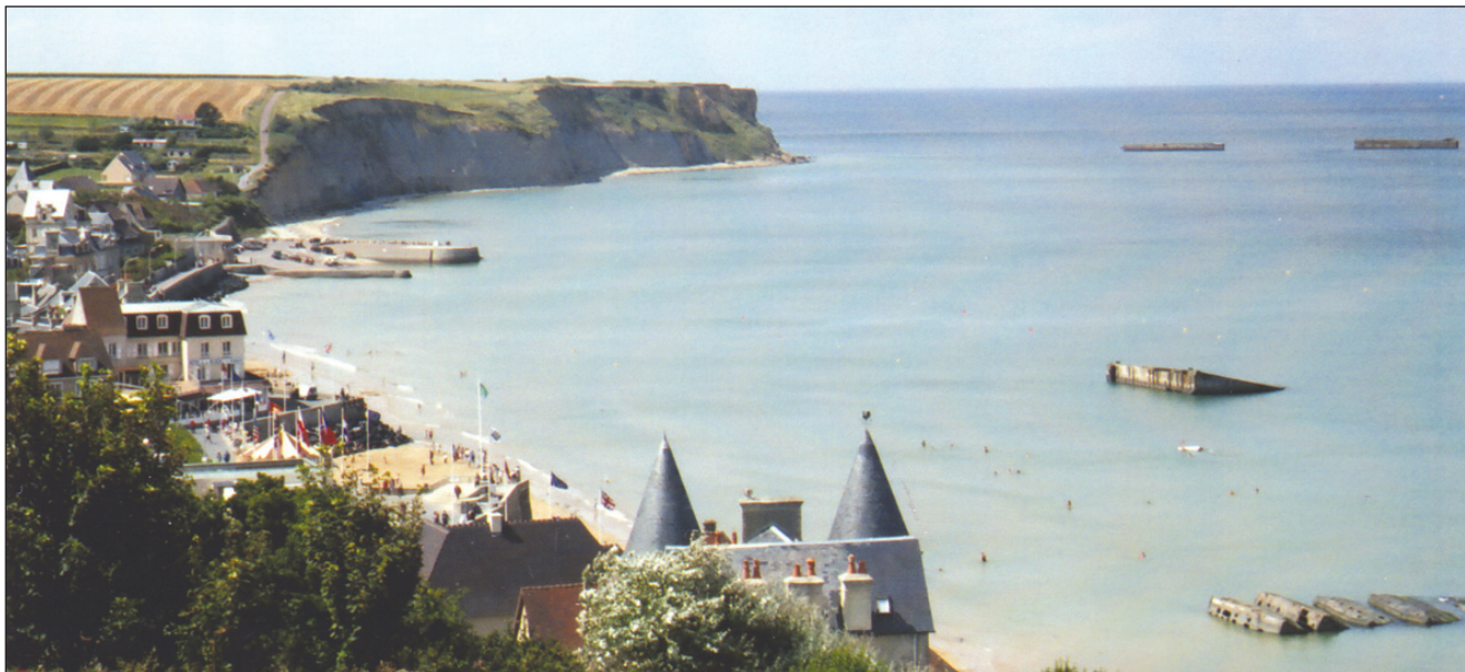
The harbour at Arromanche, Normandy in France looks very peaceful today but bears a few reminders of the Allied invasion in 1944. In the water are remnants of the prefab concrete structures used to create a safe harbour for landing craft ferrying troops and supplies.
