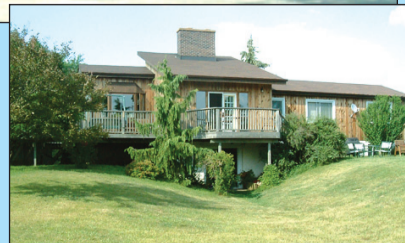
FINISHED WALKOUT BASEMENT
