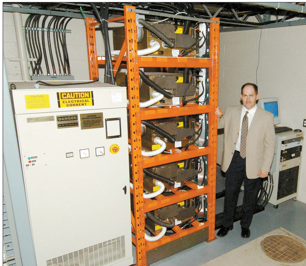
Halton Hills Hydro Inc. is launching an energy storage project this week that uses large ZEBRA batteries, shown here with the utility's president Dan Guatto, to store electrical energy bought at non-peak nighttime hours to be used throughout peak daytime hours.
