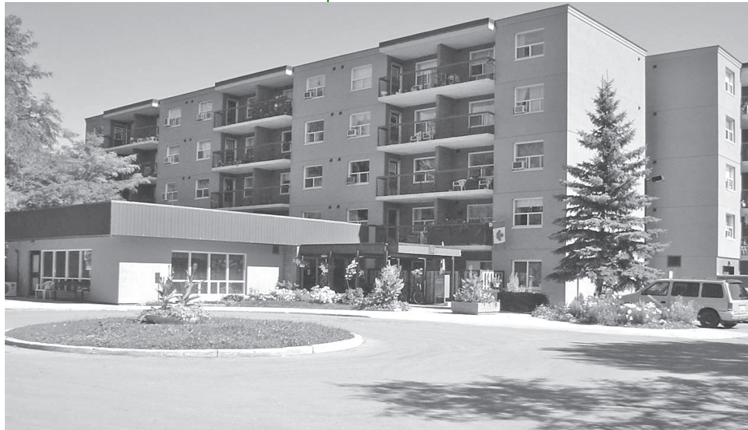
John Armstrong Terrace, affordable housing in Halton Hills.
