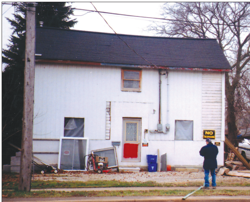
This is how the house at 52 Confederation Street looked prior to the Town of Halton Hills demolishing it last week. The Town contends the owners were given numerous chances to repair the home, but failed to meet a number of deadlines.
