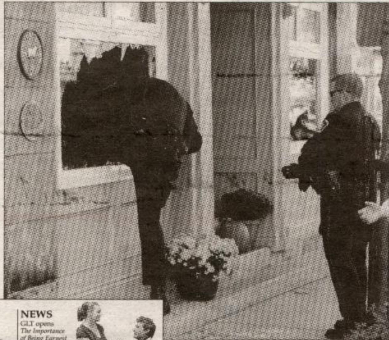
A Halton Regional Police officer climbs through a broken window at The Shepherd's Crook pub on Main Street in downtown Georgetown moments after a deer smashed through the window Saturday afternoon. The injured deer (left) was humanely destroyed by officers.
