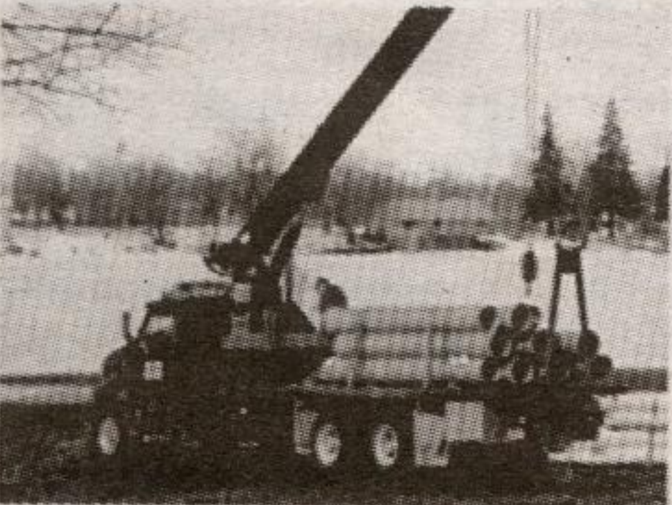
Water found! Workers bring in the Not-So-Big Pipe to Acton's Fairy Lake. The lake is expected to supply the town with water in an effort to speed up development.
