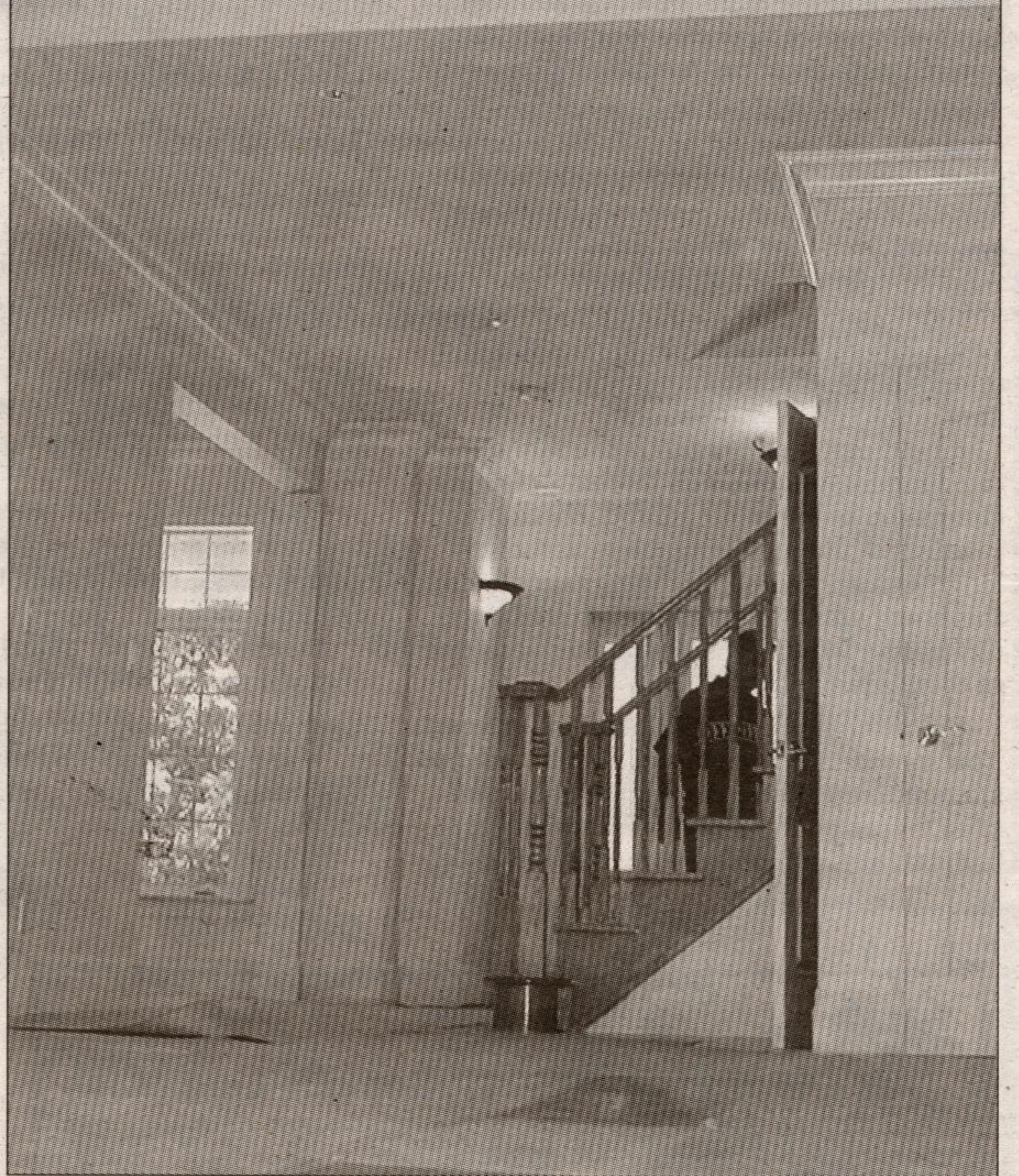
Mississauga high school students helped build this Norval home with the help of trade professionals. It was the first project of the Educational Construction Ltd. designed to introduce and train students in the building trades. Herb Garbutt photo
