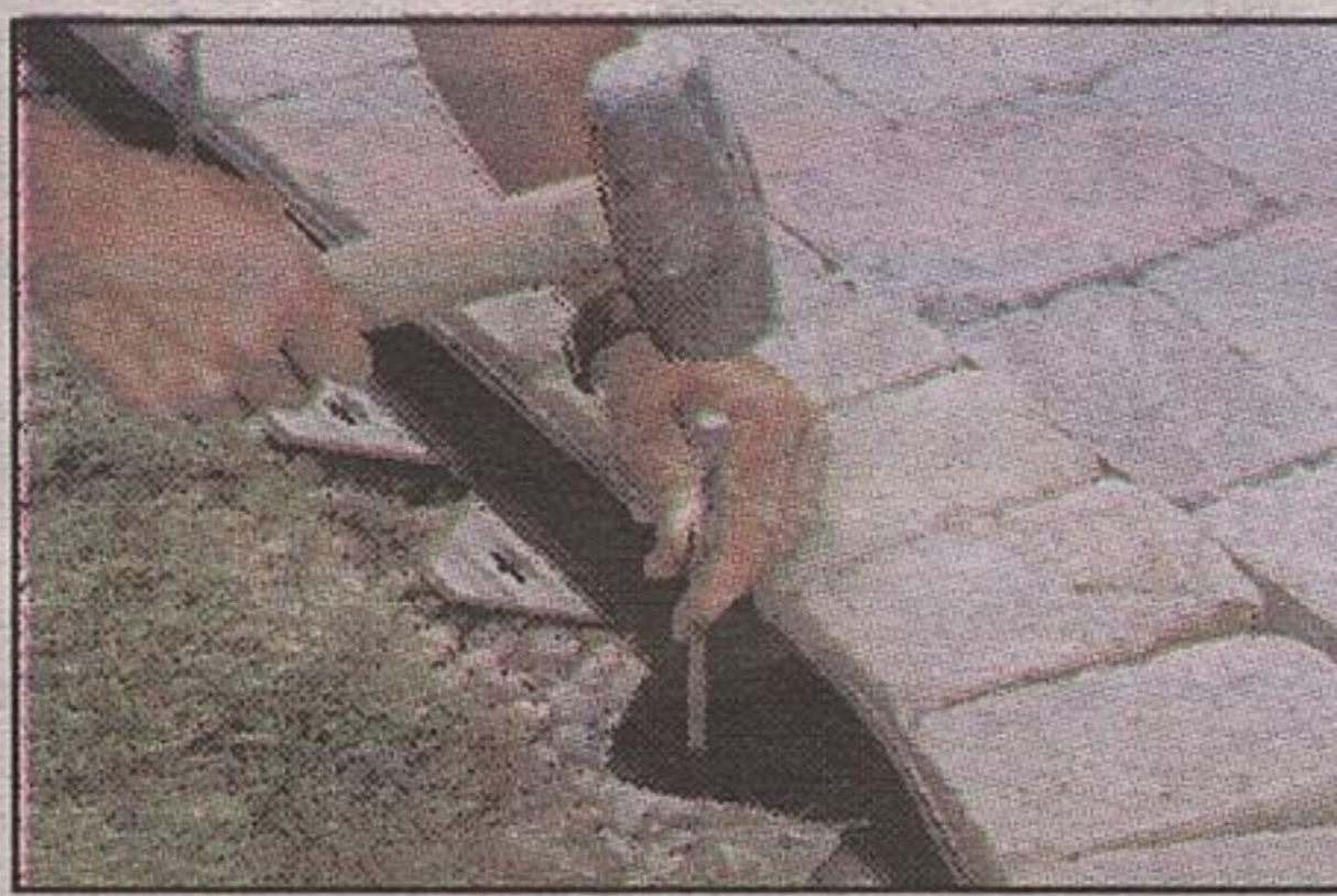
STEP 8: Edging is critical
