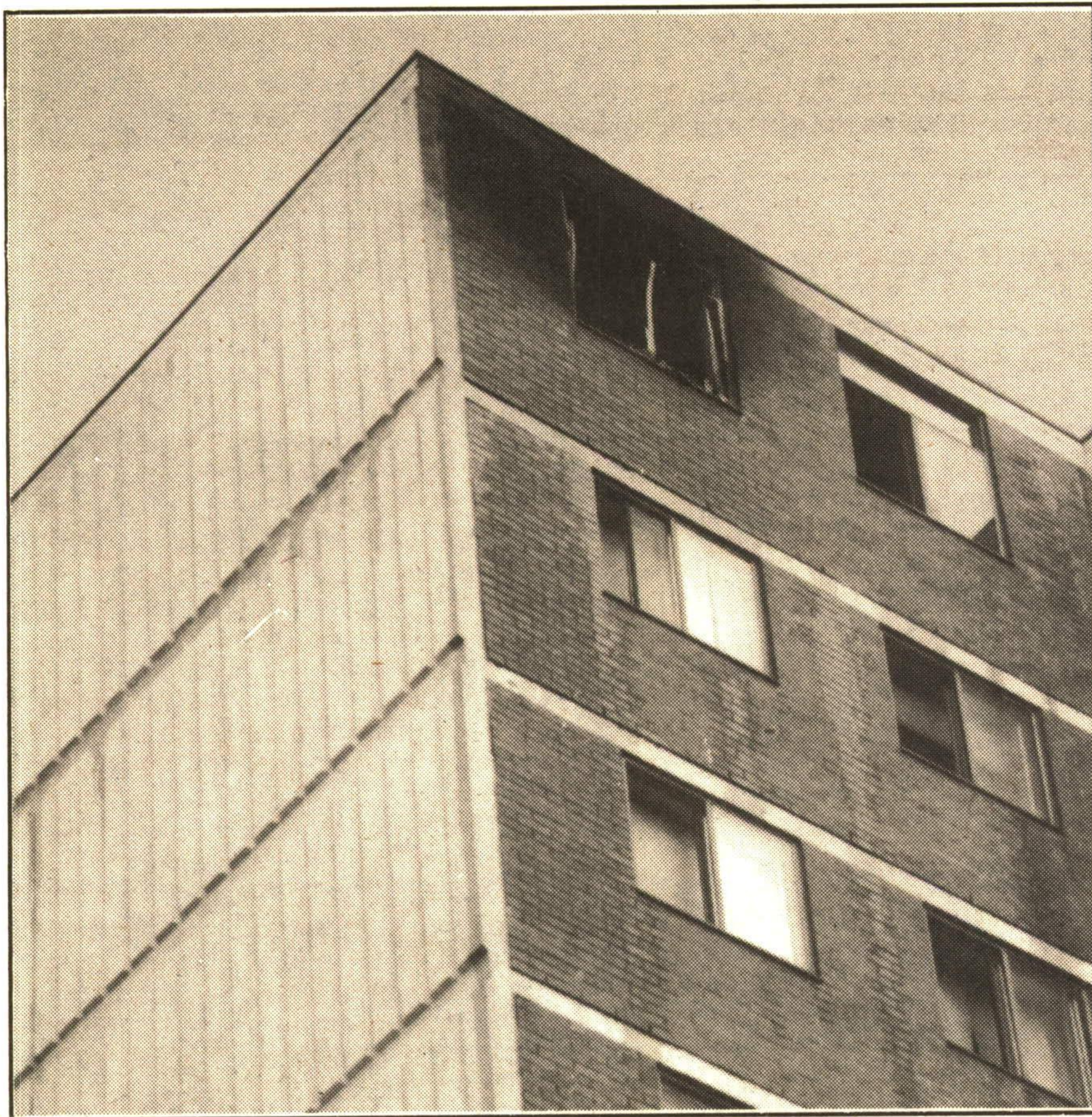
Smoke billowed out of Apartment 1101 at 60 Park Avenue, where an unattended halogen lamp is suspected of starting a fire Thursday afternoon. No one was injured, but damage is estimated at $40,000.
