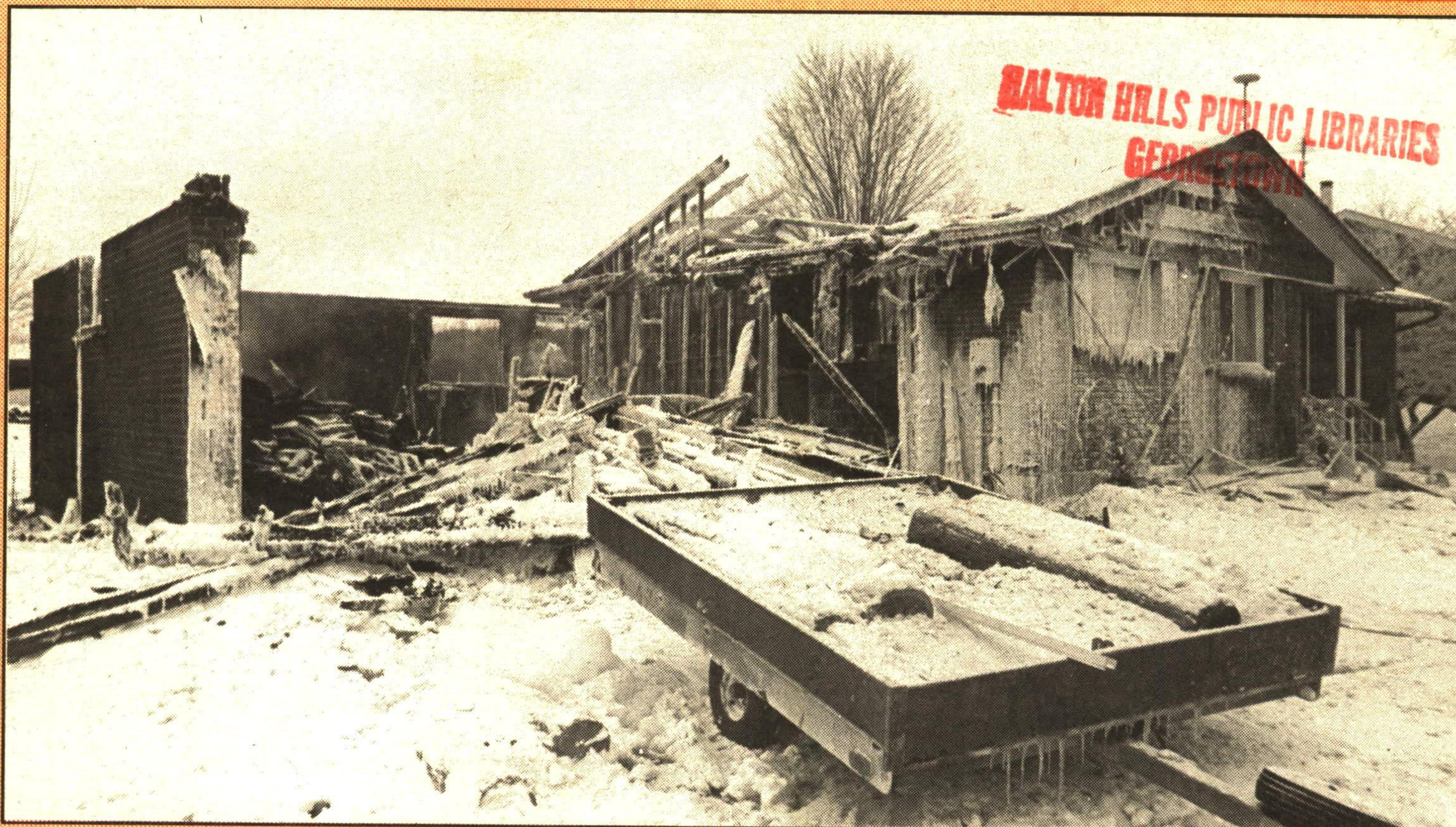
Ken Hurren and his two sons were left homeless after a Wednesday morning blaze which gutted their Third Line property, causing an estimated $200,000 damage. Donations are being accepted at the CIBC in Acton as well as the Halton Hills Hydro office, where Hurren works.
