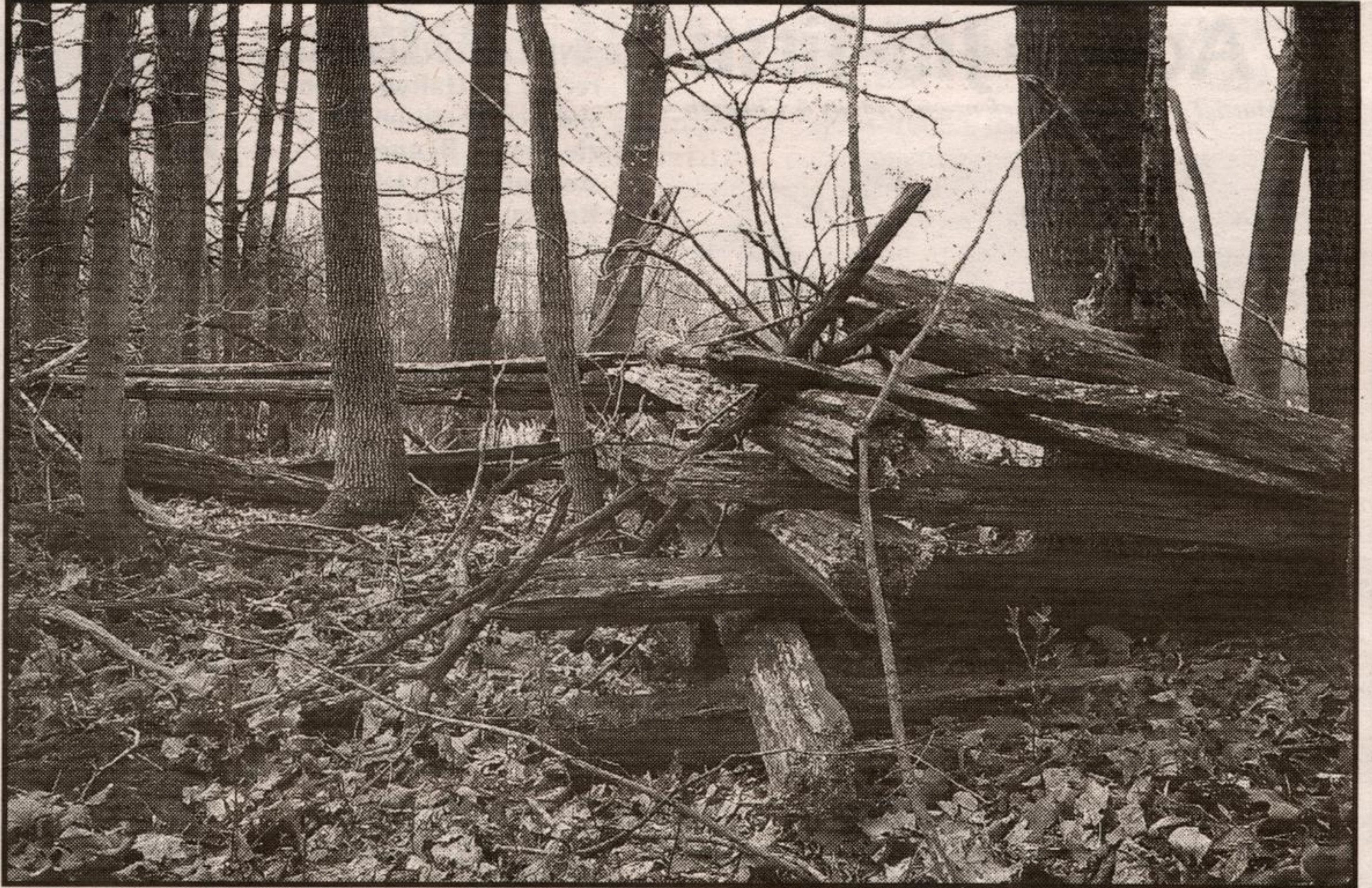
Split rail fence: Once they were as common as outhouses but few of the split rail fences which once crossed this neck of the woods are left. A legacy of the pioneers who hacked their way through the Esquesing bush, the rails kept livestock in and helped to keep some predators out. Danielle McIsaac caught this specimen of weathered cedar fence in her lens near the old Nassagaweya/Esquesing border.
