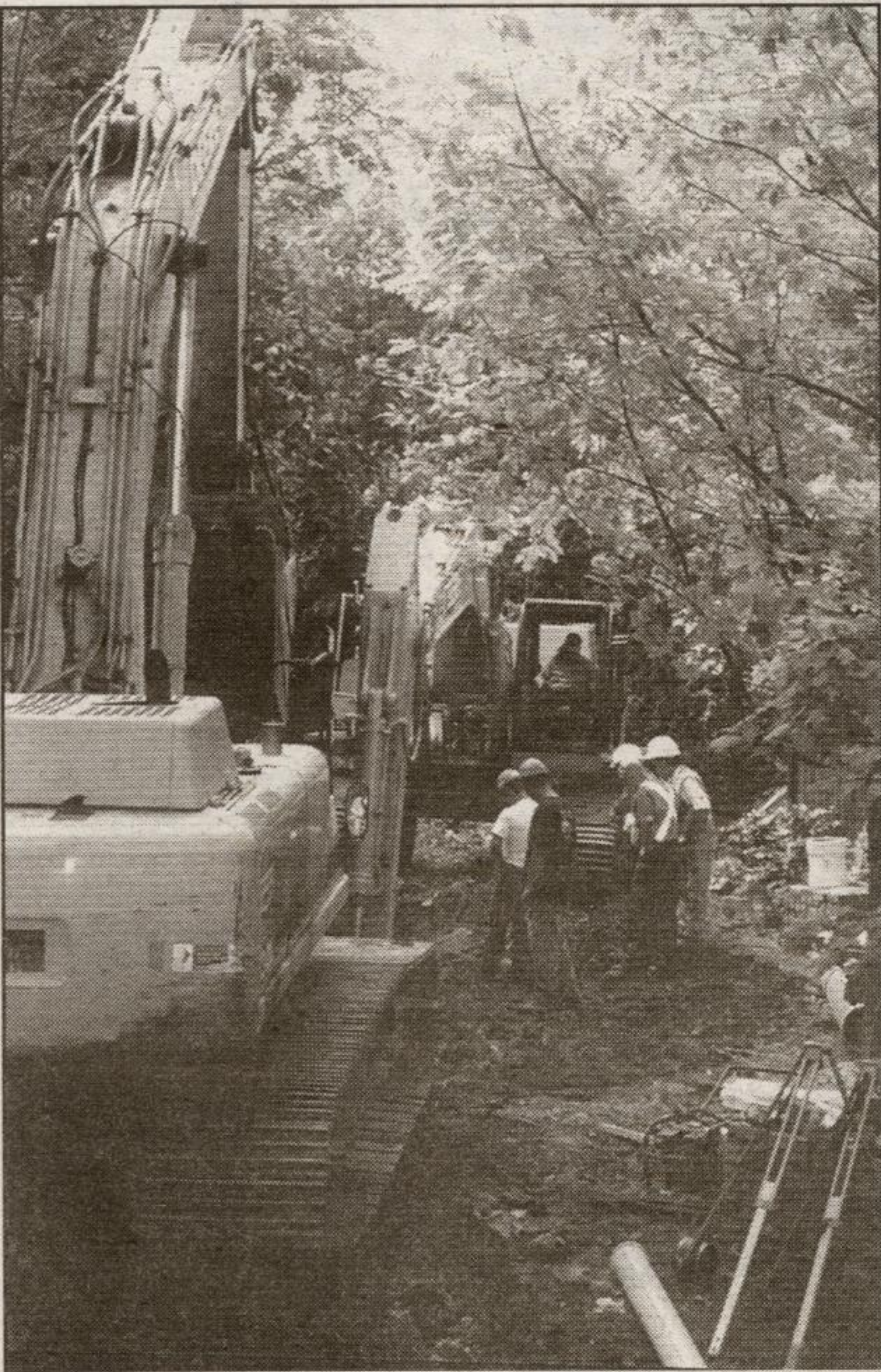
HARD AT IT: Construction crews were busy replacing fill with clean sand preparatory to starting to pave Rockwood's main street next week. Meanwhile high hoe operators with a bevy of supervisors and observers work on opening the trench along the Manse easement between Main and Carroll Streets to replace the sewer and water service. Barring complications, crews expect to begin the repaving by the end of next week. — Maggie Petrushevsky photos
