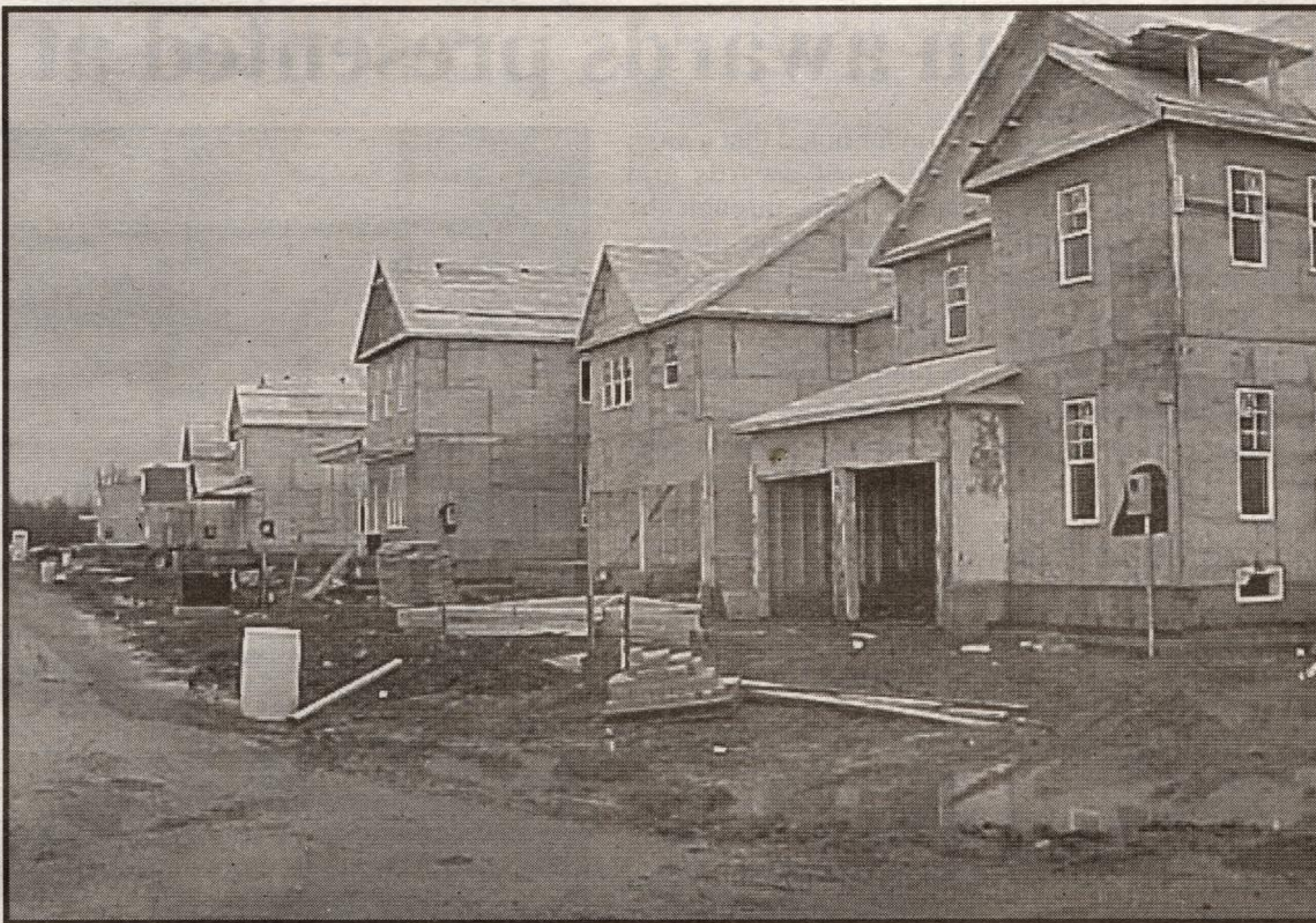
These houses weren't here a week ago.
