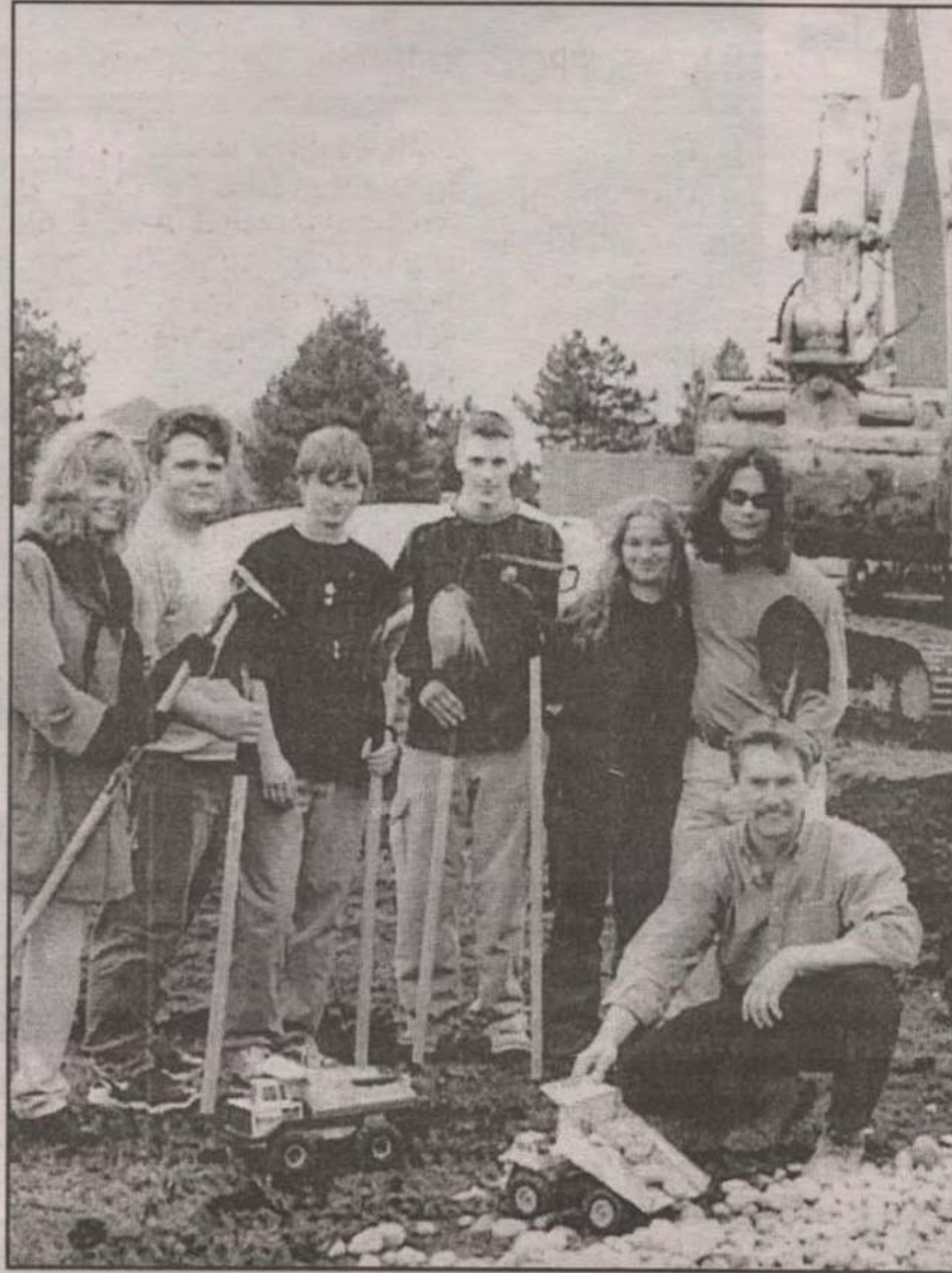
REHAB PROJECT: Acton High School students and staff were on site last week as the earthmovers began the work. They were, left to right: Instructor Sharon French, Dave Coles, Ian Douglas, Ben Elliott, Sarah Rosenmeier and Spencer Chew. Instructor Terry Roesch. — France Niblock photo
