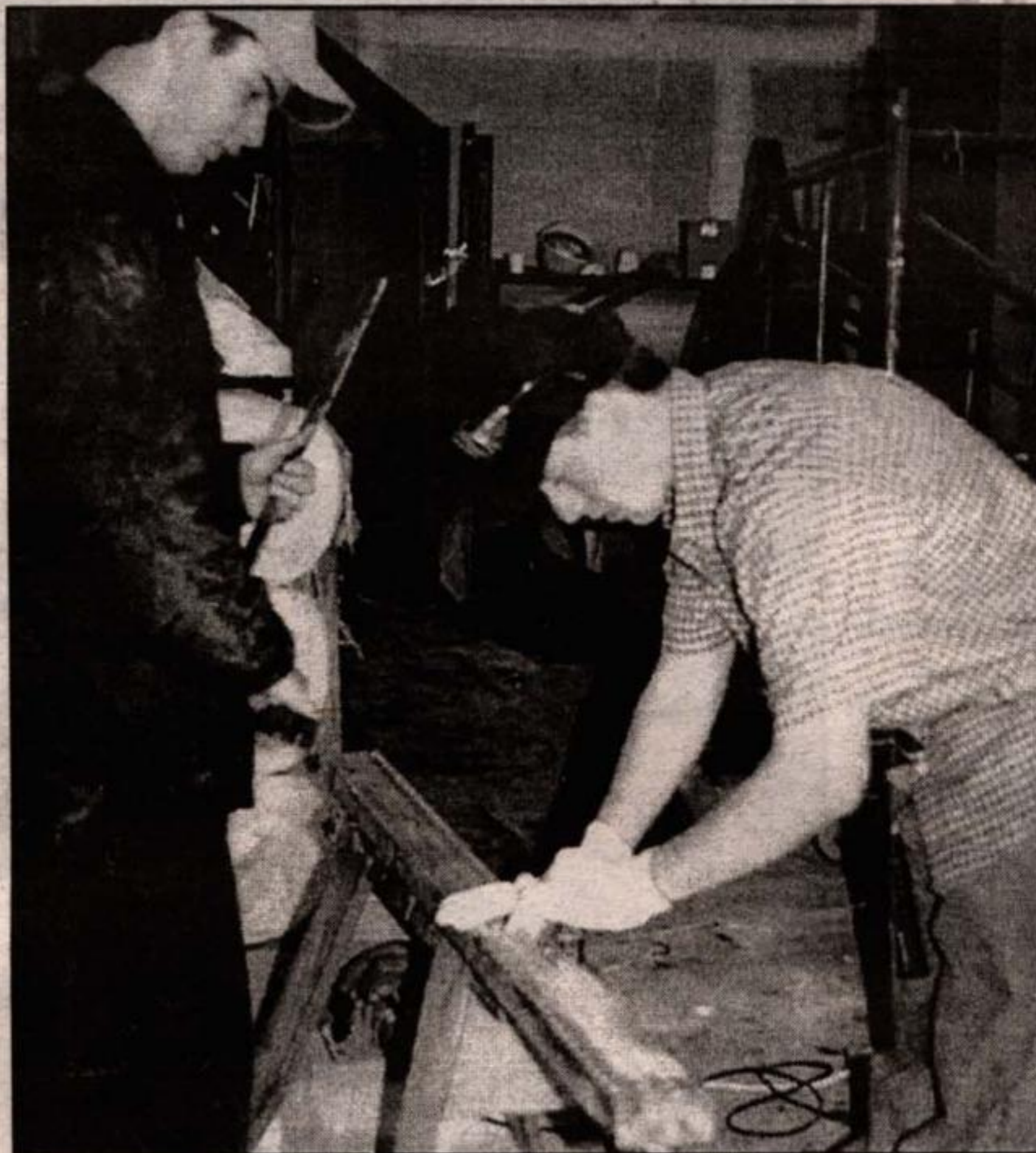
GETTING IT RIGHT: Craig Foster, left and Dave White were among 18 Gr. 12 construction technology students at Acton High school who built the new interior for the Youth Centre on Mill Street East. The class pre-fabricated walls in the school shops according to plans prepared for the Youth Centre and installed them on site Friday. - Maggie Petrushevsky photo
