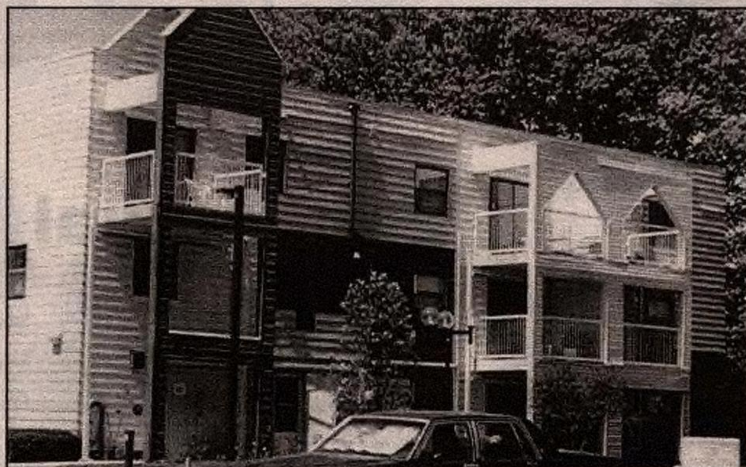
FACELIFT: The Squires Lodge, Rockwood's senior apartments, will receive new cladding, new windows, new doors and work on its balconies. The lodge board has received a provincial grant to cover the cost of the improvements.
