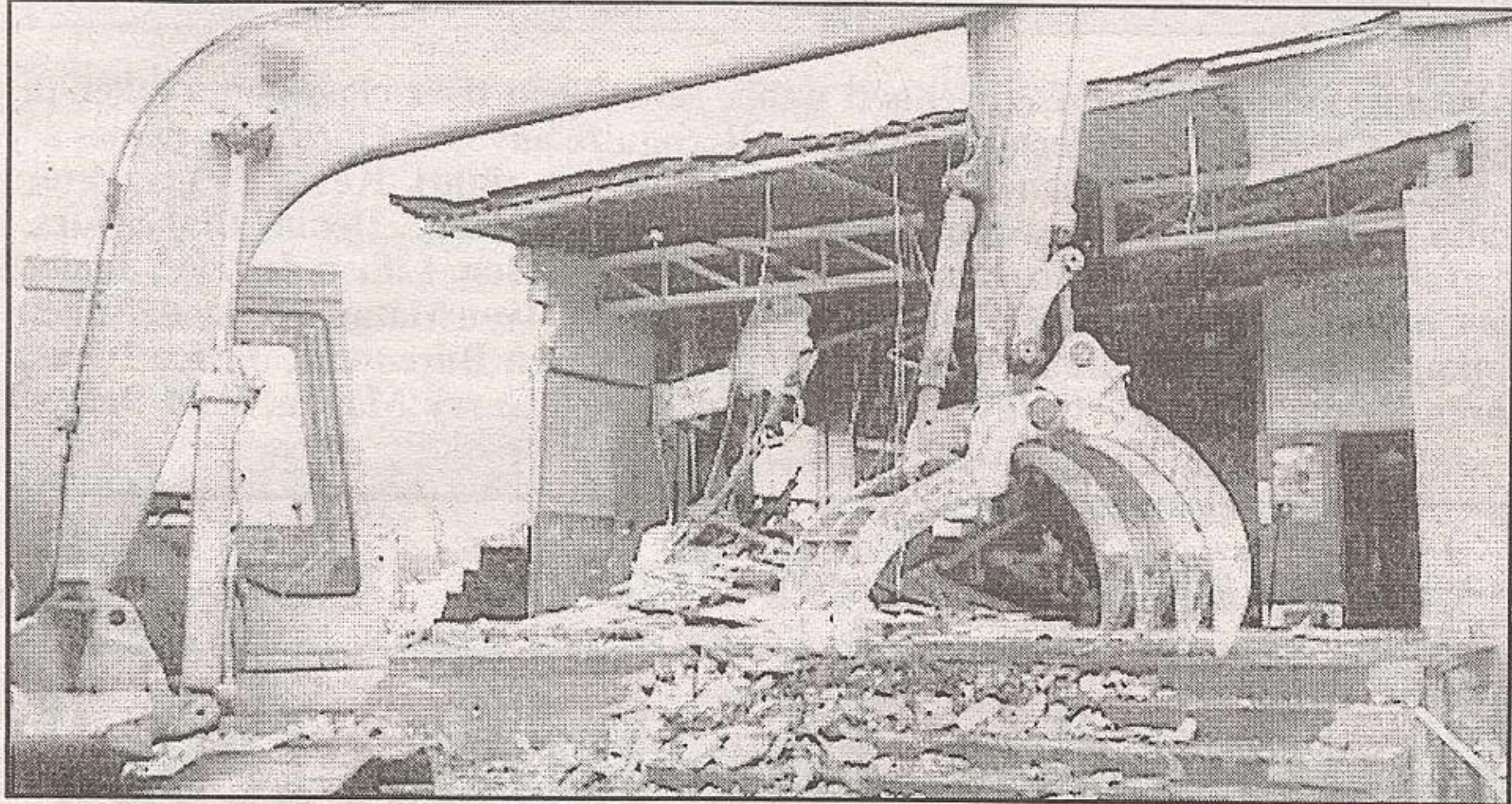
NO MORE HOCKEY HERE: The inside rink area of the arena is being stripped of the side boards. Above the rink, a crew is in the process of removing all the roof panels and fasteners...more than 10,000 of them. While below, the front entrance to the old arena was torn down in a matter of hours. Blocks, glass and steel that once housed the seniors centre was being loaded into dumpsters. - Angela Tyler photo
