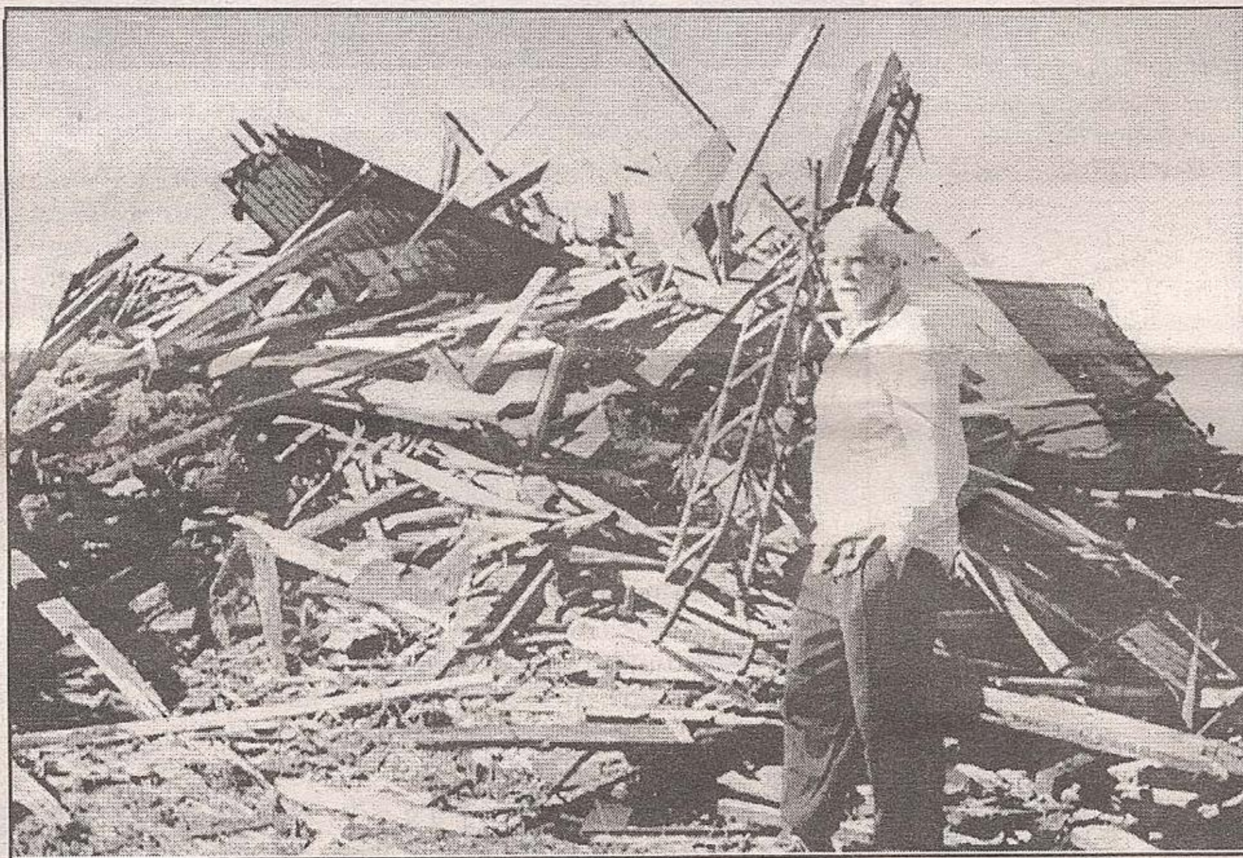
CLEANUP CONCERNS: Acton Boulevard homeowner Henry de Vries is concerned about the fire and safety hazard posed by this pile of debris behind his home. - Frances Niblock photo
