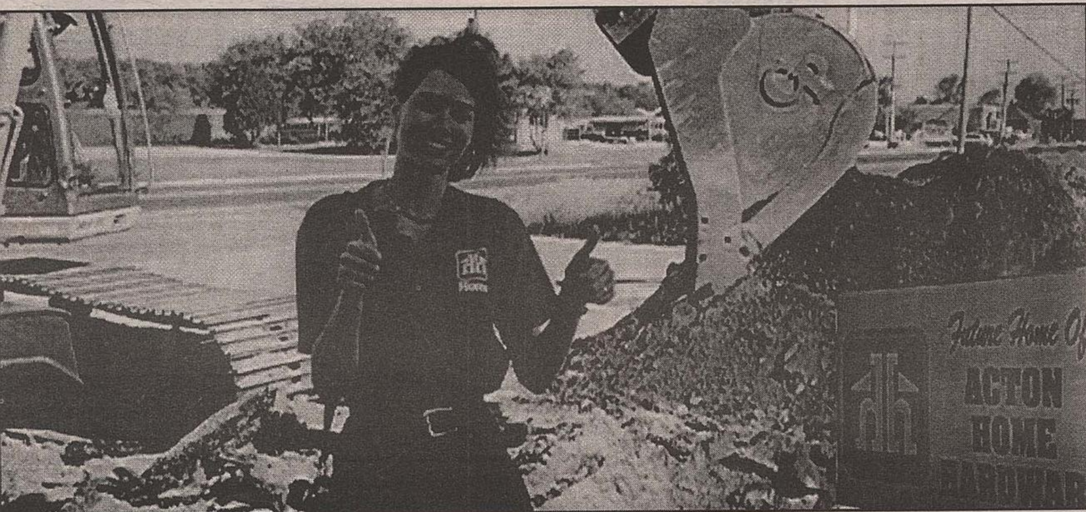
TWO THUMBS UP: Acton Home Hardware's Val Manes gives her approval to the construction that has started at their future home this week on Queen Street East. — Ted Tyler photo
