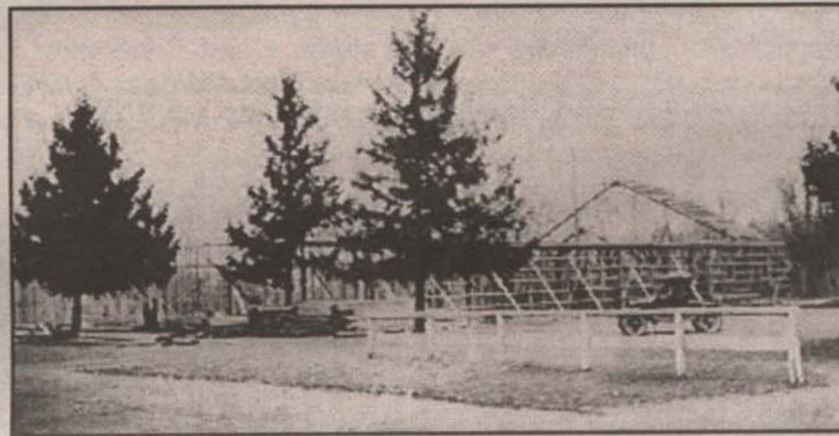
The building of the old arena on Oct. 20, 1929. - Photo submitted by Bob Landsborough
