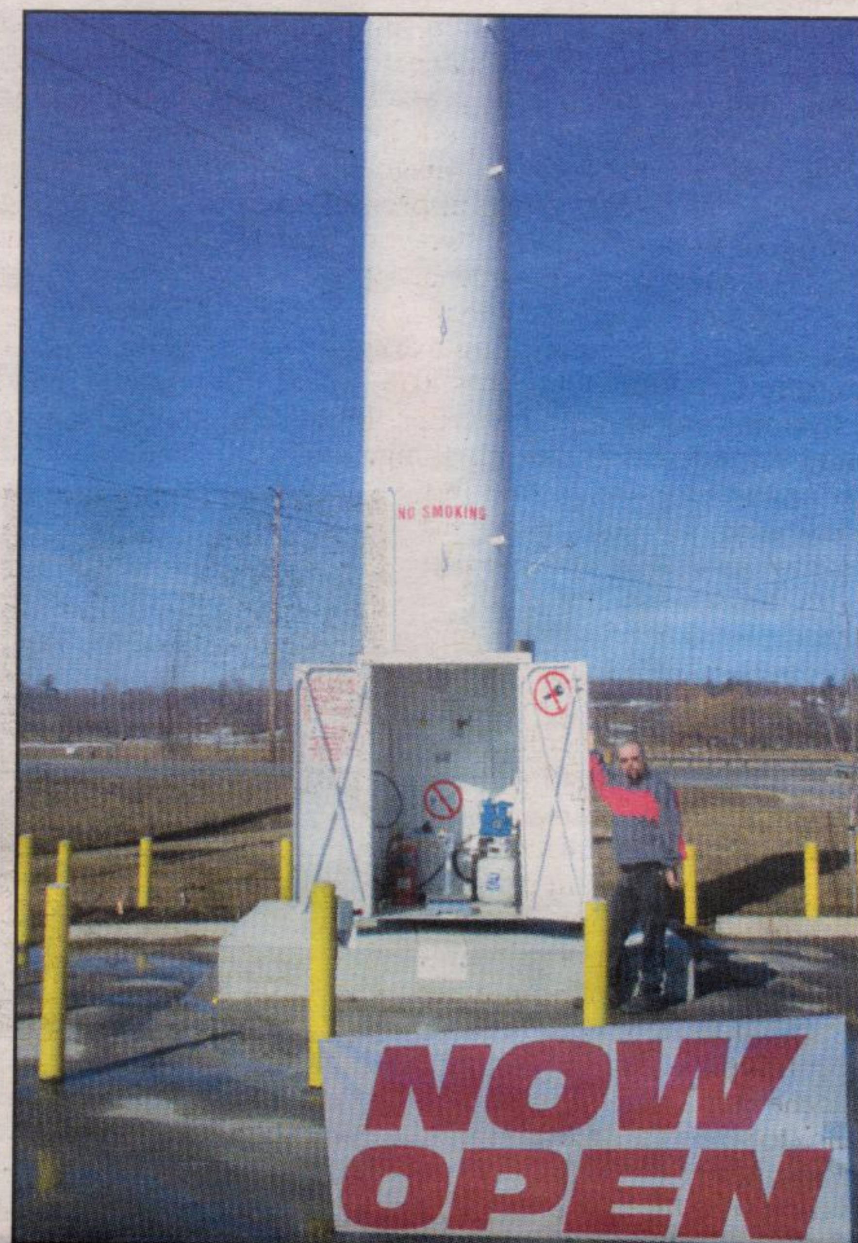
Rob Paris pictured with his new propane tower ready for lift off.
