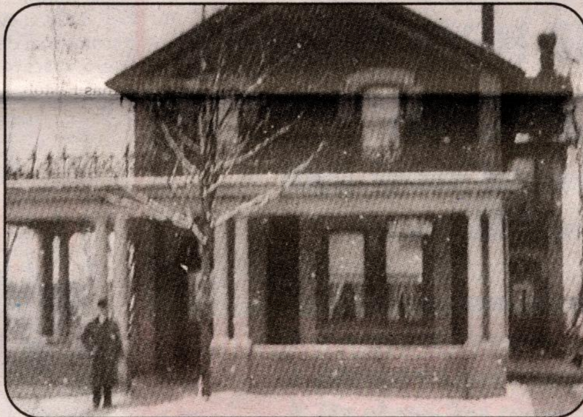
Uncle Johnny's Boarding House 289 Woolwich Street, Guelph ~ circa 1920 ~
