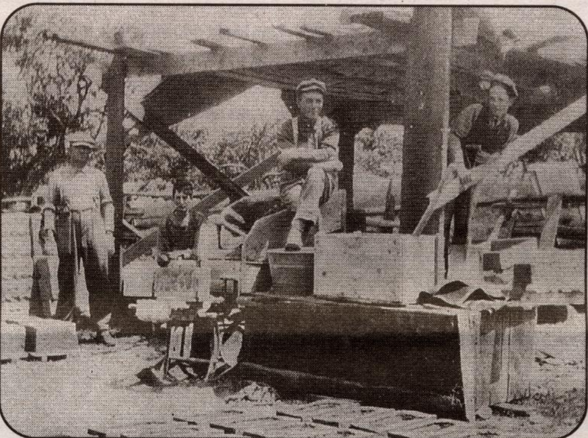
George Watson with sons Milton & Siebert making cement blocks for silo building, on Lot 32, Conc. 5, Nassagaweya in the early 1900s.
