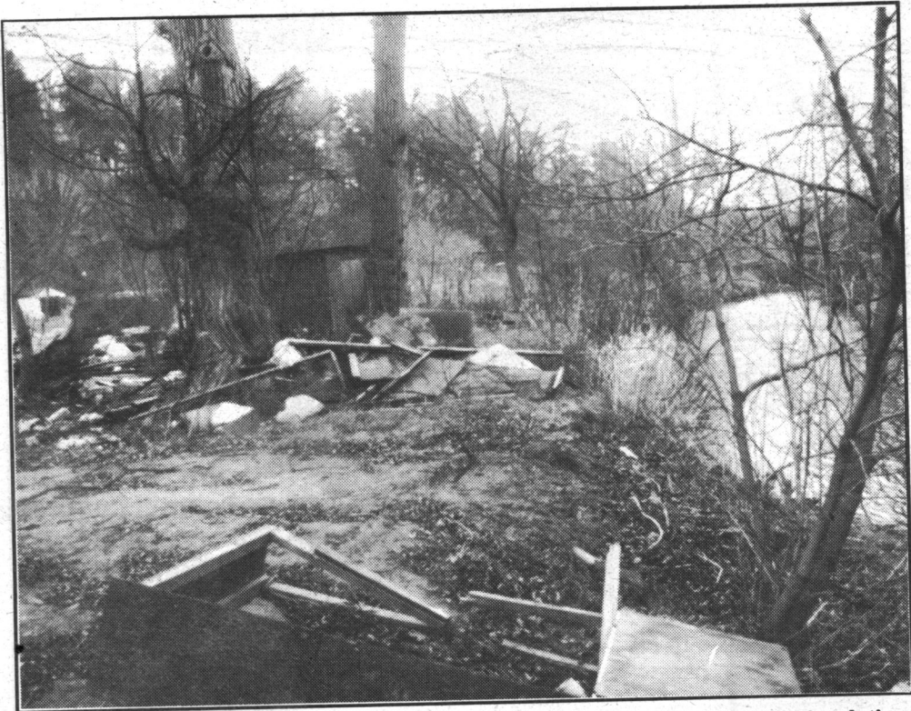
An undrained septic system, open septic wells, abandoned buildings, blowing insulation, refuse and rats have turned Willow Park in Norval into a health and safety nightmare. photo submitted
