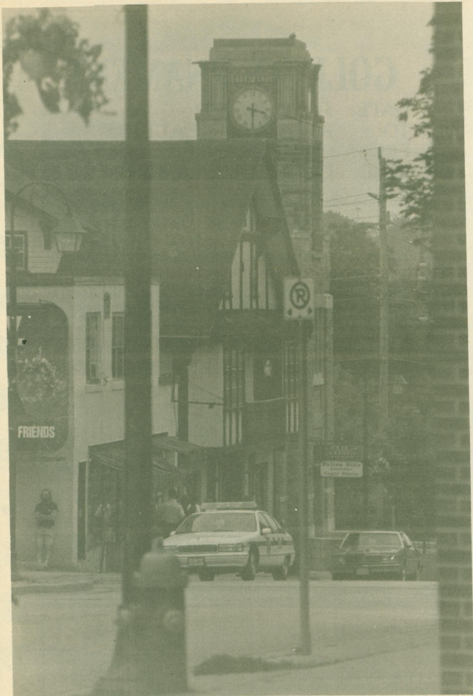
The clock tower in the old post office building on Mill Street was the object of police surveillance during a gun call Friday.
