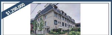
$1,298,000 ETOBICOKE OPPORTUNITY! Executive 3 bedroom freesthold townhome in prime location. Rooftop terrace with views of the City & the Lake. Quartz counters, Gas Stove & Fireplace, 3 Skylights. Lots of upgrades! Walk to the lake, parks, restaurants & public transit. Few minutes to downtown Toronto & Pearson Airport.
