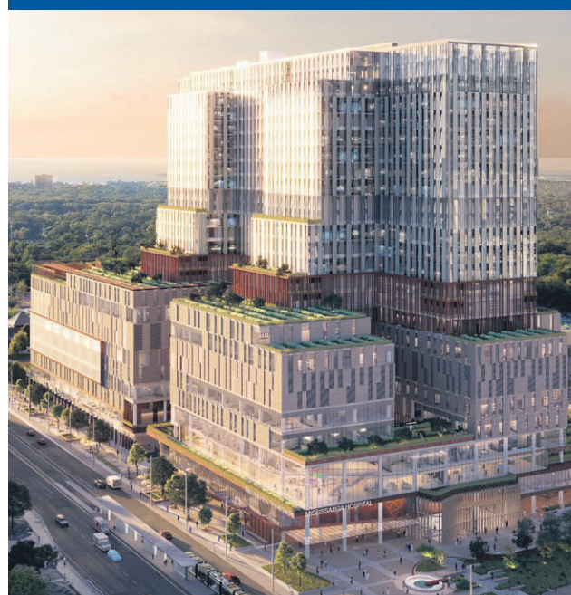
The Peter Gilgan Mississauga Hospital
