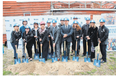
Habitat for Humanity photo Members of Habitat for Humanity Halton-Wellington-Dufferin break ground on the 37 King St. project.
