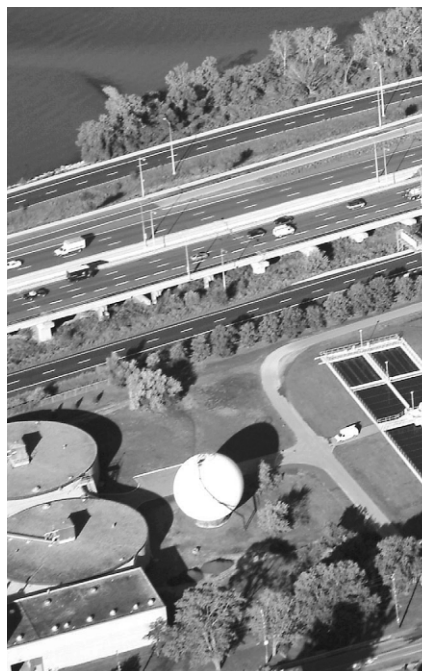
Skyway Wastewater Treatment Plant
