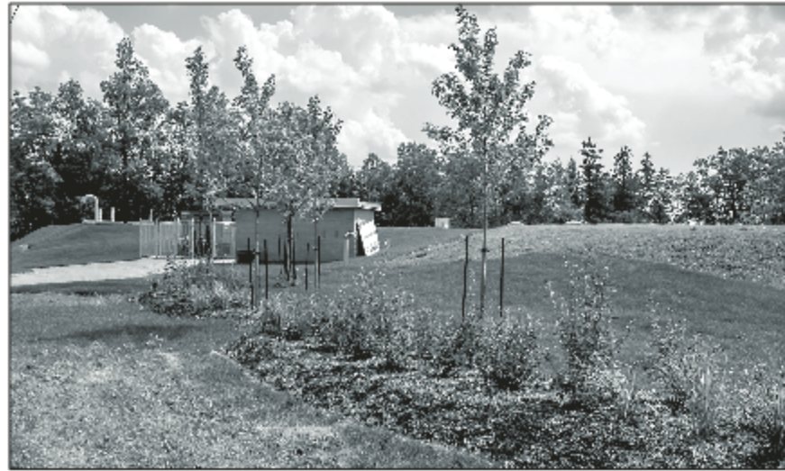
RESERVOIR GETS REVAMPED: A major expansion of the reservoir, at the top of Churchill Road North, has been completed. New grass, trees and planting beds have replaced the dirt, concrete and construction materials that dominated the site during the work. - Les Schmidt photo
