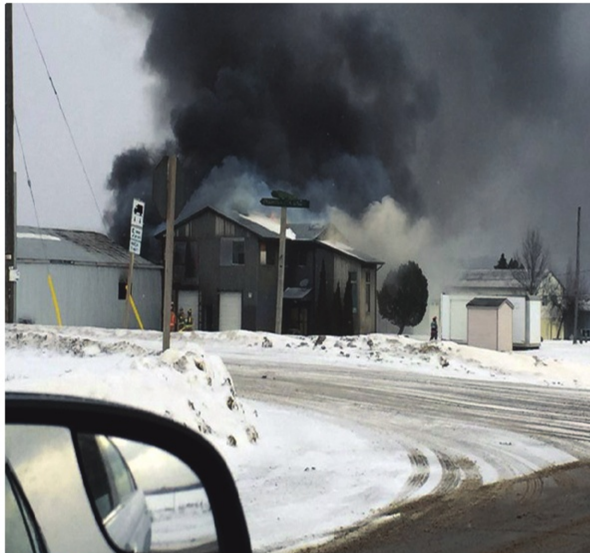
RESIDENTIAL FIRE: Hwy. 7 was closed just west of Acton for a couple of hours Monday due to a structure fire. Fire crews from Halton Hills and Guelph-Eramosa responded to a call of a blaze in a mixed commercial/residential structure at around 10:30 a.m. Ontario Provincial Police closed Hwy. 7 between Sixth Line Nassagaweya and Crewsons Corners until 1:30 p.m. There were no reports of injuries, and the fire cost approximately $1 million in damages.
