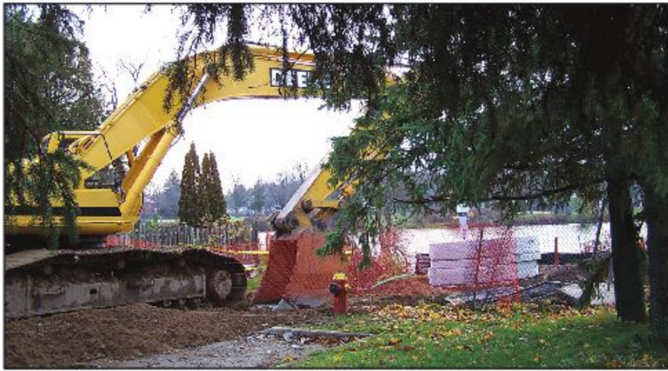
WATER WORKS: By tomorrow (Friday) the Town's installation of two water quality structures in Prospect Park should be complete. The devices, like this one at the end of Elmore Drive, and one at the end of Tyler Avenue, will clean storm water before it enters Fairy Lake. — Marie Shadbolt photo
