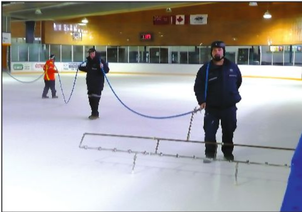
ICE MAKERS: By next Tuesday, the ice will be in at the Acton arena, ready for the first senior shinny games which will kick off the hockey/skating season. On Monday, Town employees Kyle Thomson (left), Tim Bennett and Tav Ariganello applied many thin coats of water to build up the surface. —Frances Learment photo
