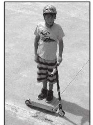
NOT THAT DANGEROUS: Acton's Brandon Miles, 10, knows to avoid this previously-repaired crack and hole at the 3-Musketeers skate park. – Frances Learment photo
