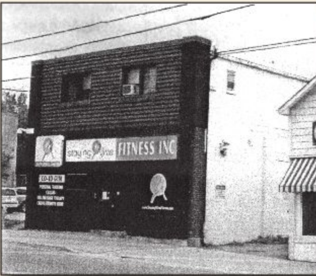
The former building of the Acton Creamery at 11 Main Street North, Acton, now a fitness studio in 2013
