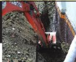
EXTERIOR EXCAVATION AND WATERPROOFING
