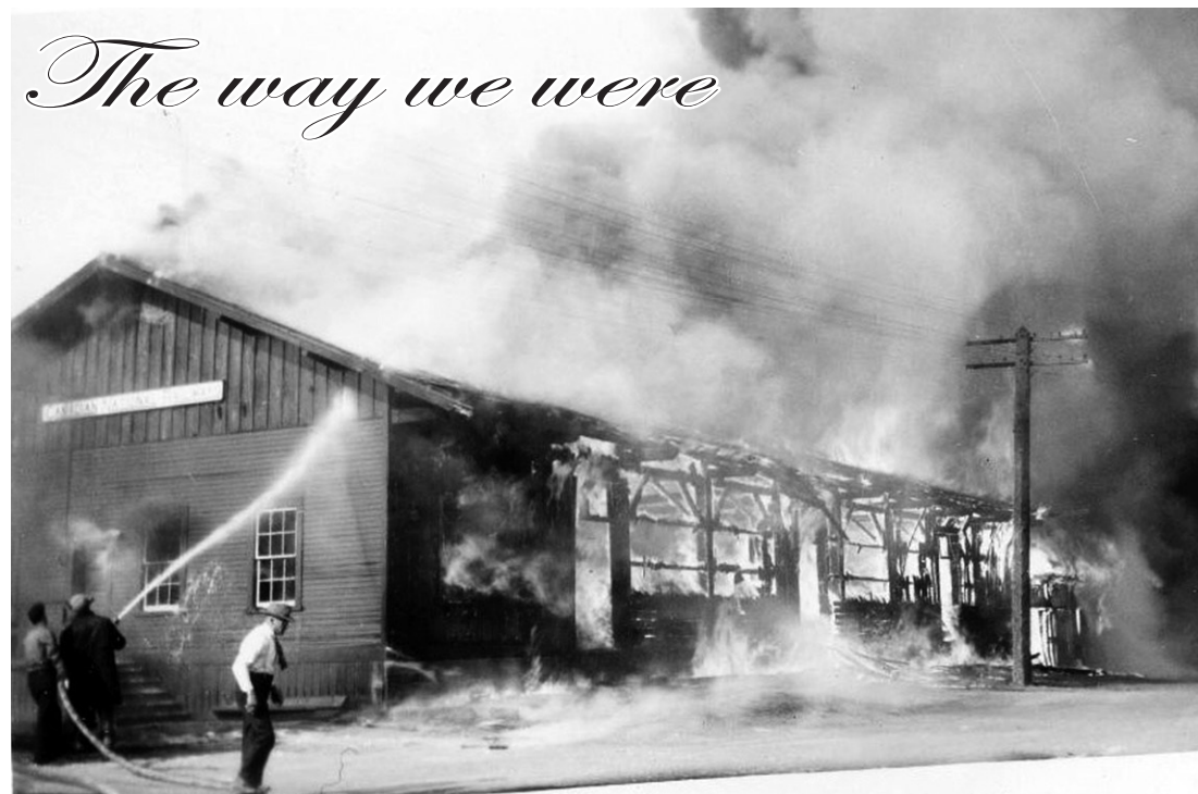
In this photo from April 22, 1946, flames wrap around the frame structure at the CNR freight yard in Georgetown. This spectacular fire destroyed the 160-by-70 foot freight sheds, three railway cars loaded with freight, the J.B. Mackenzie coal shed, and a home owned by Mackenzie, but occupied by the Tyler family that stood nearby. The blaze resulted in damages of close to $60,000.
