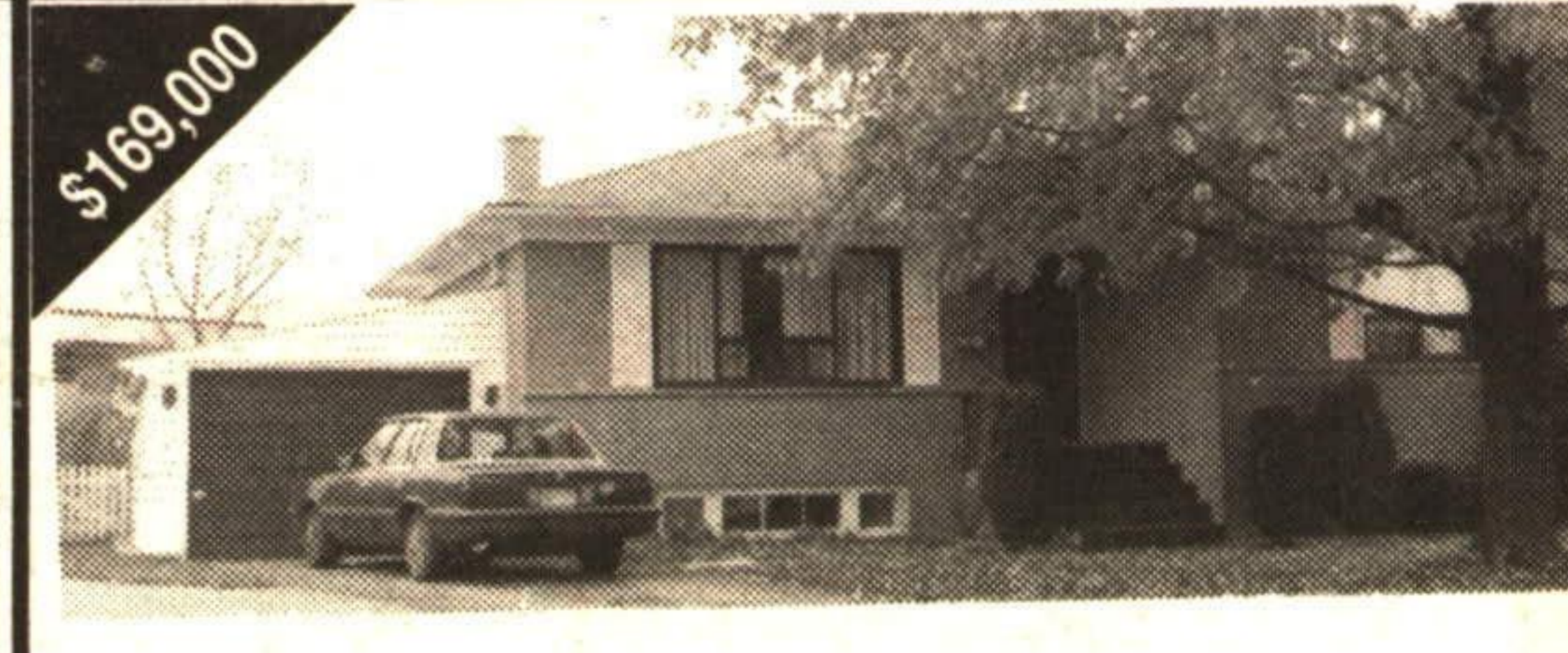
THIS SOLID BRICK HOME... has a lot to offer and its pie-shaped lot is situated on a cul-de-sac, many features, new windows, C.A.C., finished rec with fireplace and more...Good home for only $169,900. Make the call today 873-3377. Ask for Yvan*. CW93-040
