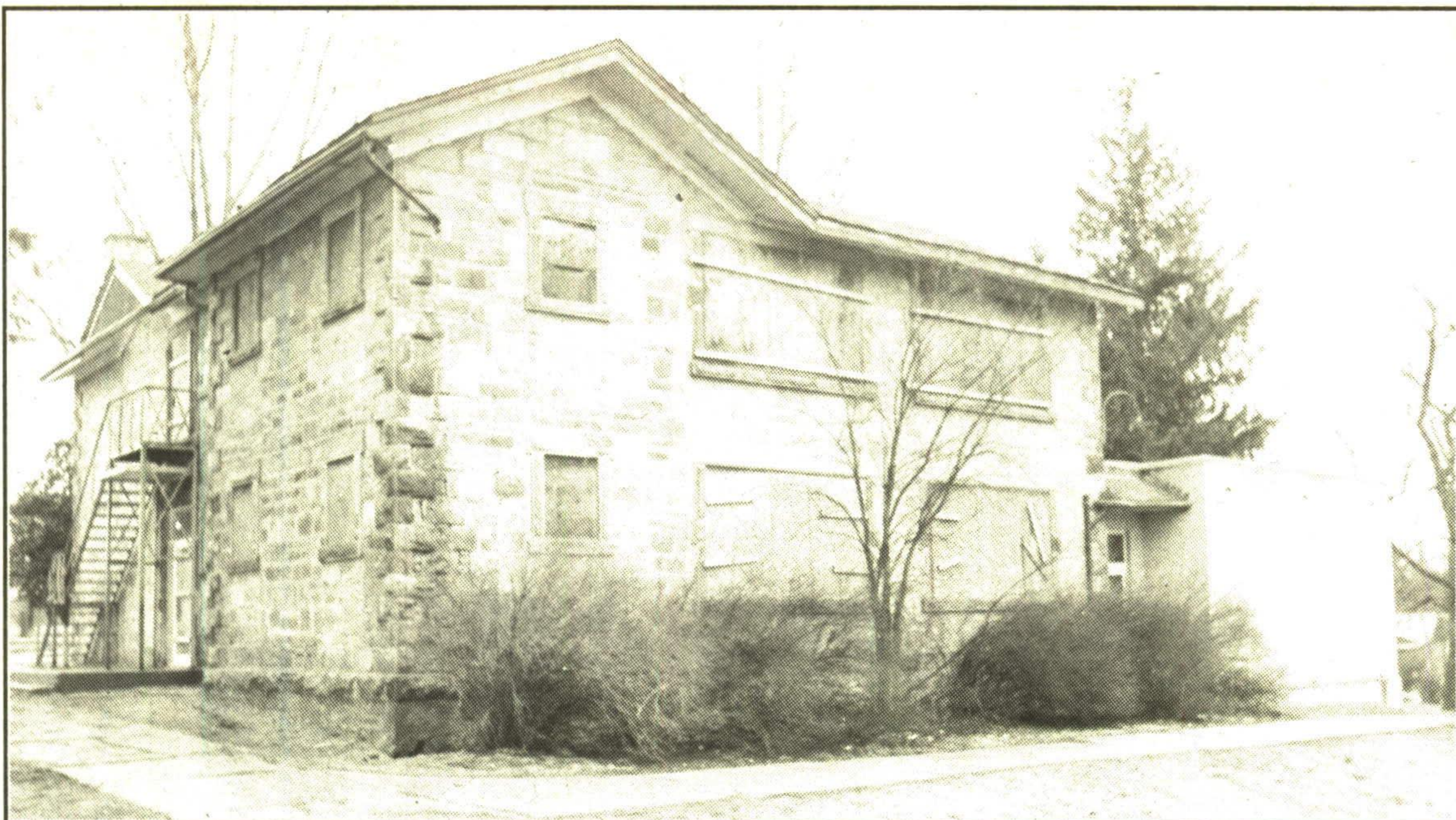
An Acton group, the Local Architectural Conservation Advisory Committee (LACAC) is attempting to meet with Halton Board of Education officials to discuss the fate of this old schoolhouse, which dates back to 1925.
