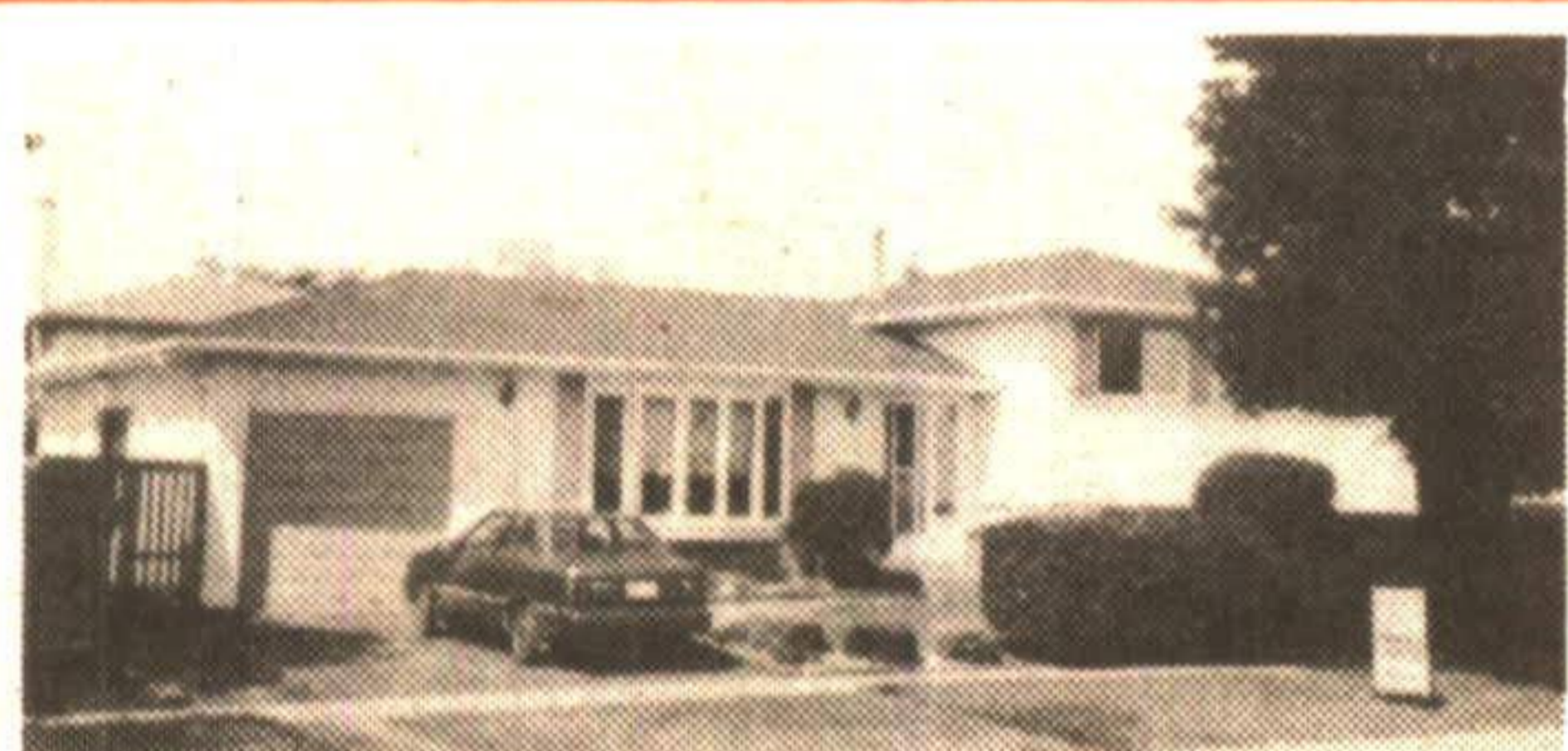
POOL - UNDERGROUND SPRINKLERS
