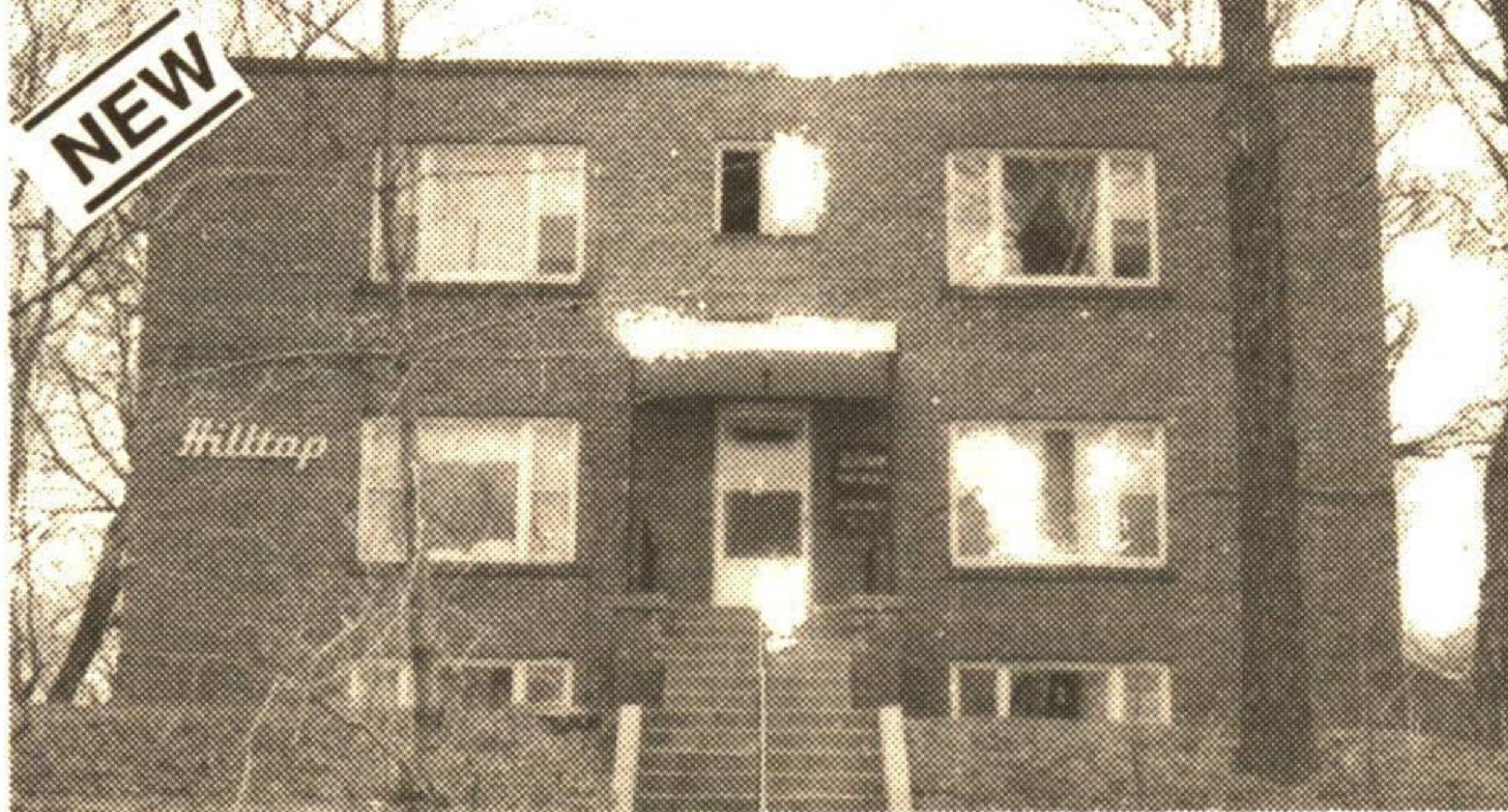
15 UNIT APT. BUILDING IN GEORGETOWN
