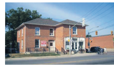
RENOVATED COMMERCIAL/RETAIL UNIT $1,150/Month
