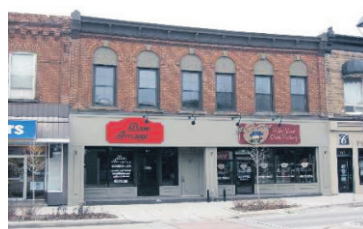
BRAND NEW 2ND FLOOR OFFICE SPACE $1,600/Month 12-033 W2277844 www.haltonhomes.com
