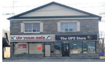
LOCATION! LOCATION! LOCATION! $2,300/Month
