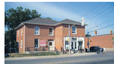
RENOVATED COMMERCIAL/RETAIL UNIT $1,150/Month
