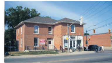
RENOVATED COMMERCIAL/RETAIL UNIT $1,150/Month
