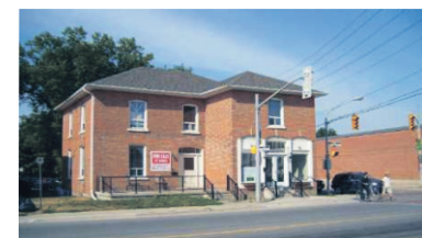
RENOVATED COMMERCIAL/RETAIL UNIT $1,150/Month
