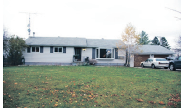
2+ AC, GARAGE/WORKSHOP W/HEAT & HYDRO $415,900
